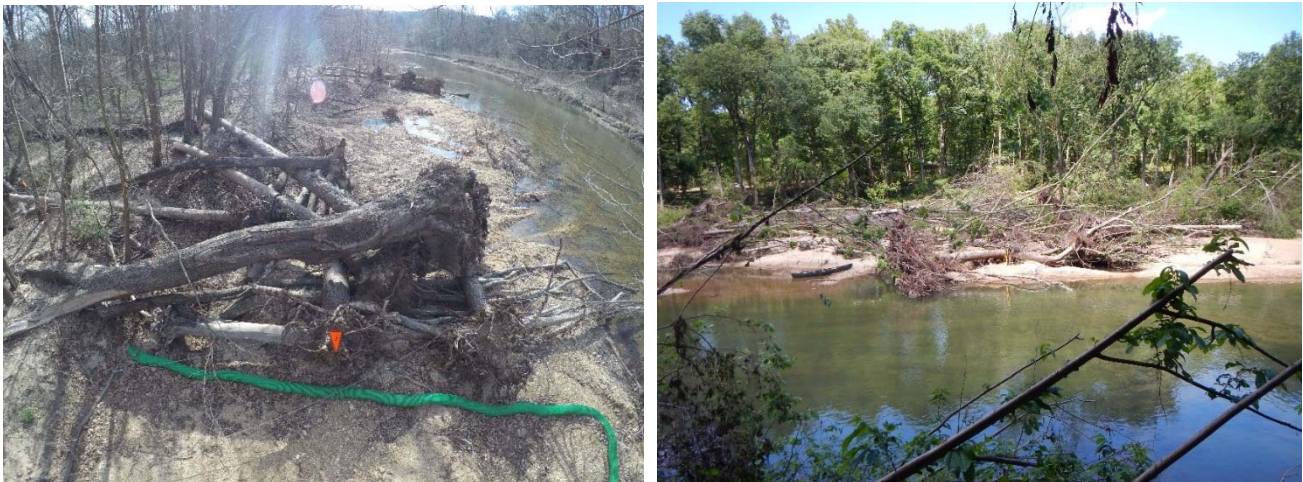
Figure 16 - Left photo is a lateral bar jam constructed on the North Fork White River in Missouri to store sediment and recruit wood to control sedimentation from a campground. Left photo is the log jam structure pre-flood, the Right photo is post flood photo. Note the large accumulation of logs and sediment on and adjacent to the log jam. Accumulation was more than 3ft deep of sediment.
