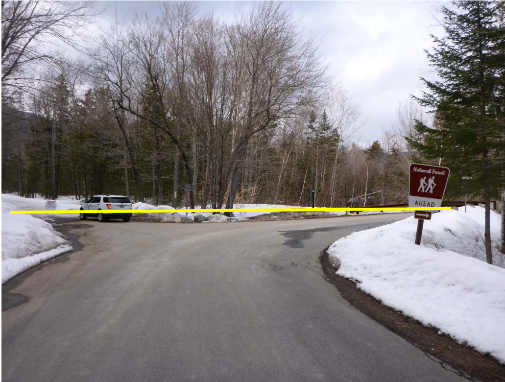
Figure 10 - Tripoli and Livermore Road junction at the avulsion location. This view is downstream looking upstream at the junction. Raise the road grade to ~ the yellow line. Install the largest pipe arch or elliptical pipe possible under the Livermore road while maintaining 18" of cover on top of pipe or to manufactures recommendations. Construct a flood channel to the river from the outlet of the pipe.
