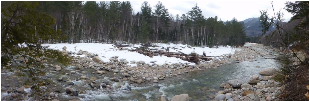
Figure 1 - View upstream of the impacted trail/road section looking downstream at the depositional bar and log jam forcing the river into the river right bank along the trail
