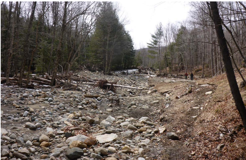
Figure 15 - Channel section downstream of the large alluvial fan on Tunnel Brook. This section of channel is accumulating wood and aggrading sediment.
